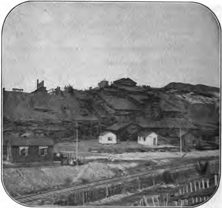
FIG. 92.—A large building is required to prepare anthracite coal for market and the earth is encumbered with refuse. Eastern Pennsylvania.
